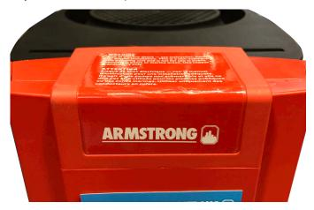
**Step 3:** Remove screw securing the fan cover as shown. Remove the fan cover from the pump.
